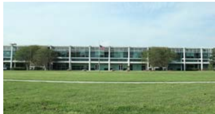
Baton Rouge Recreation & Parks (BREC) Administrative Offices
