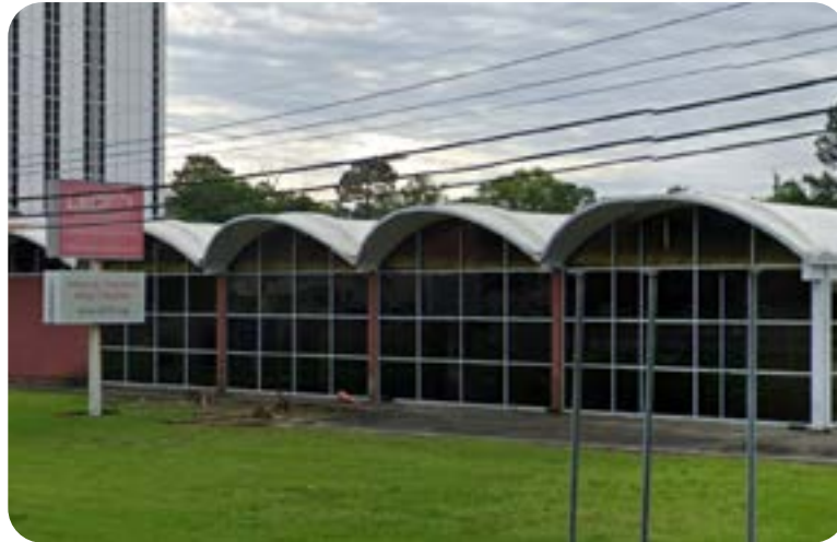
3.1 5550 Florida Blvd, LA Resource Center
